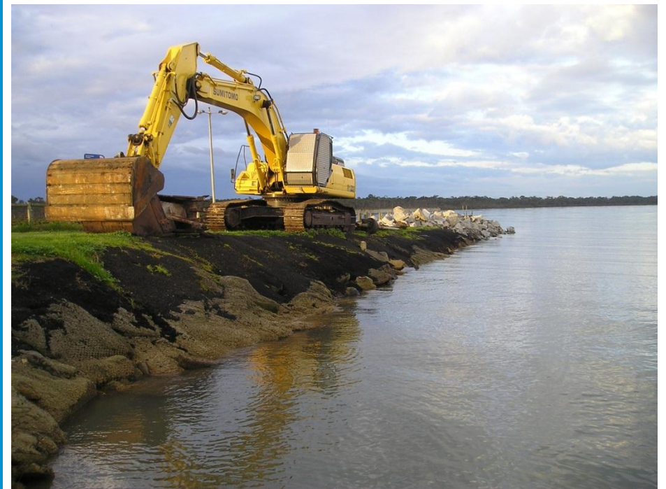
Figure 38: Ongoing maintenance and emergency repairs costs associated with ‘business as usual’ need to be factored into the assessment
