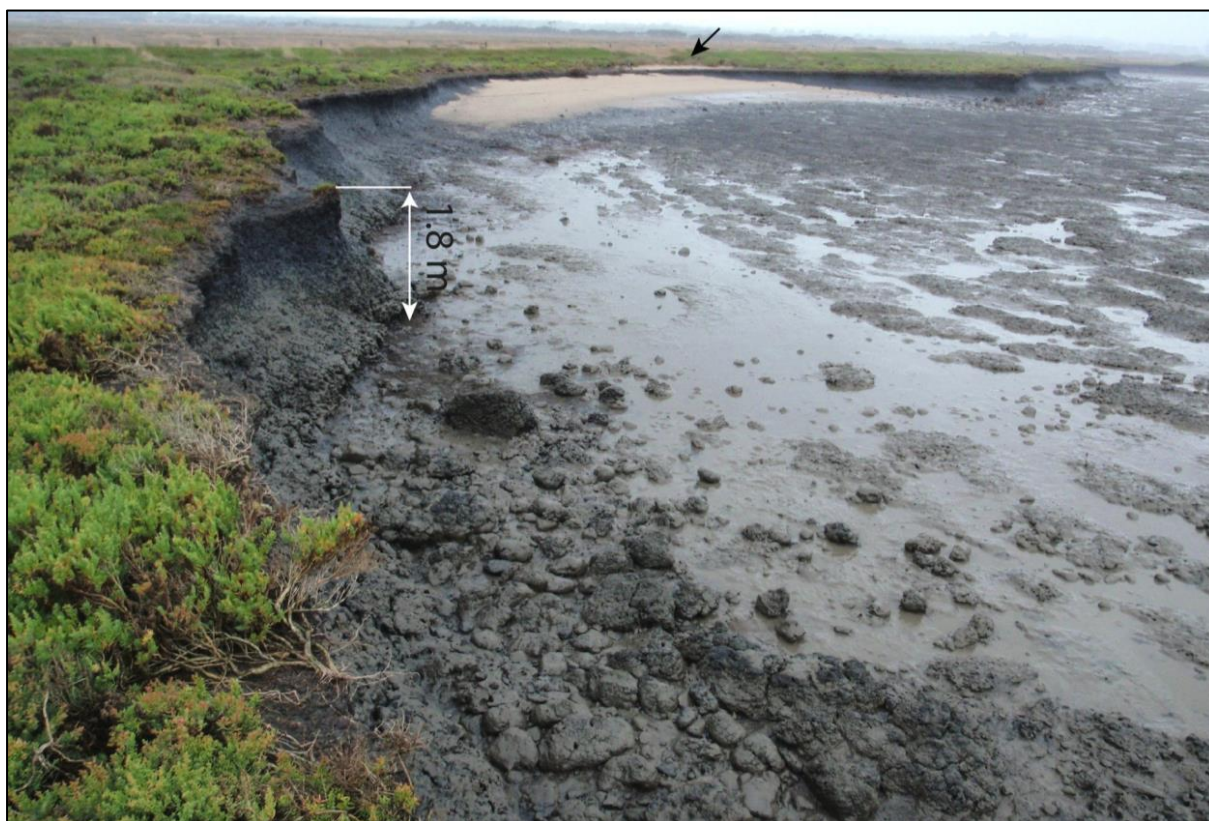
Figure 4-5 Sand in Embayment and Cliff Base South of Lang Lang River ( the arrow shows the chenier of sand and shell at cliff top )
