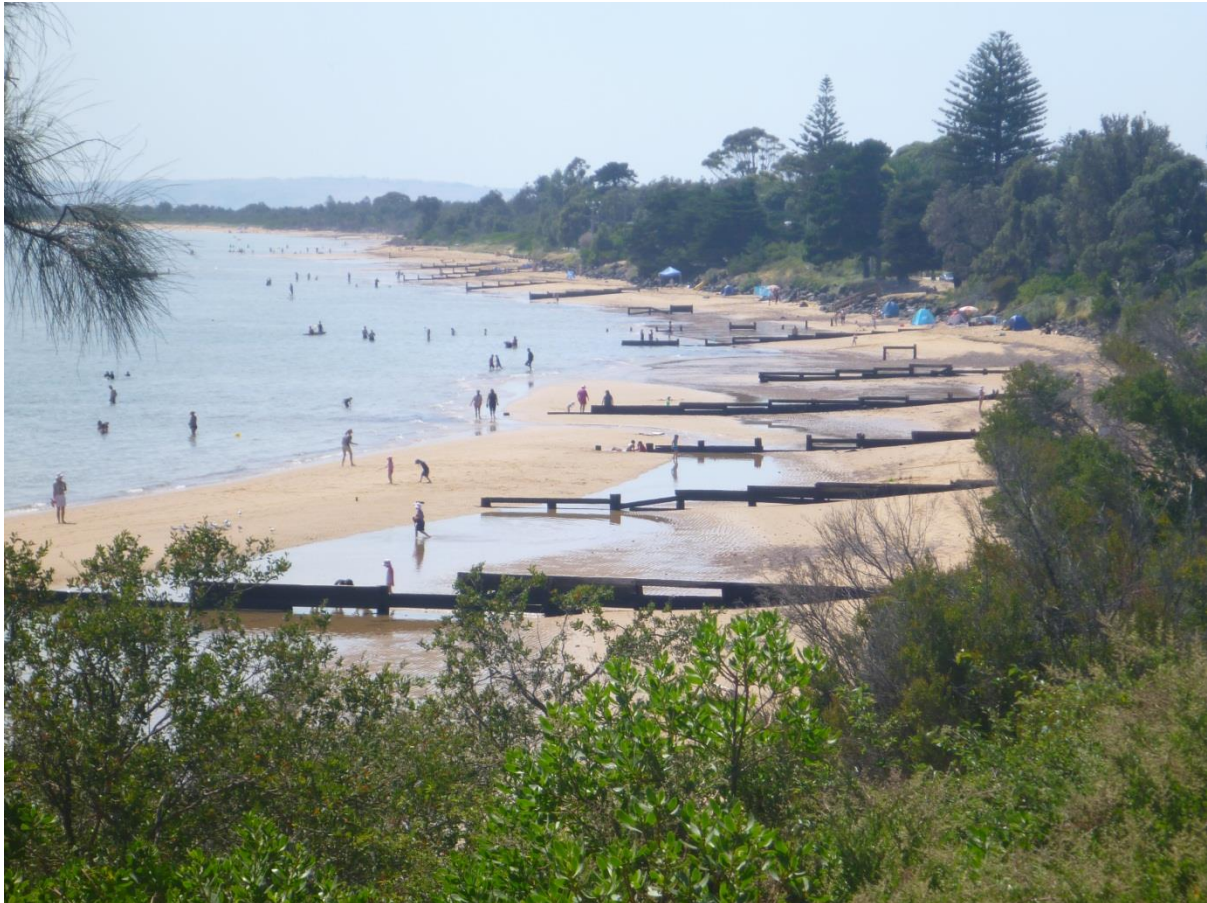
Figure 5-7 Timber Groyne Fields, east of Erehwon Point in January 2014
