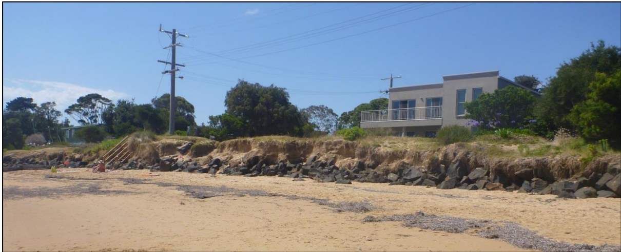
Figure 5-8 Example of rock revetment along Silverleaves shoreline
