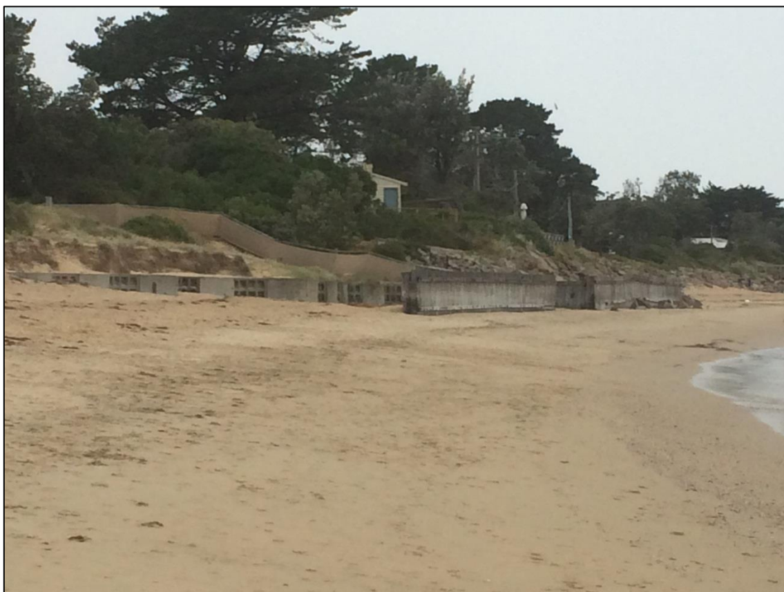
Figure 2-14 Sections of Private Sea Wall at Somers
