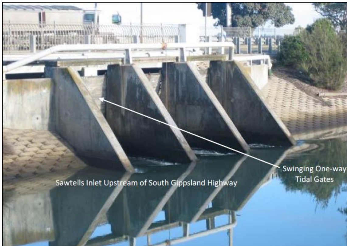
Figure 3-9 Sawtells Inlet Tidal Gates
