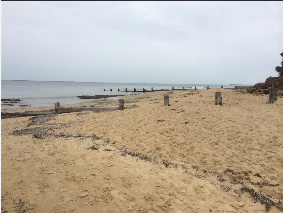
Figure 2-10 Timber Groynes at Balnarring Beach
