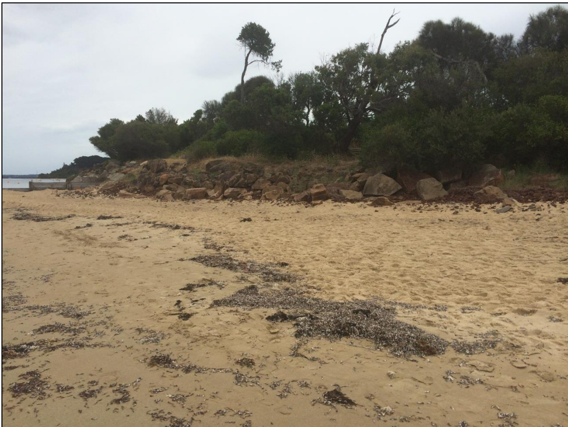
Figure 2-11 Rock Revetment at Balnarring Beach
