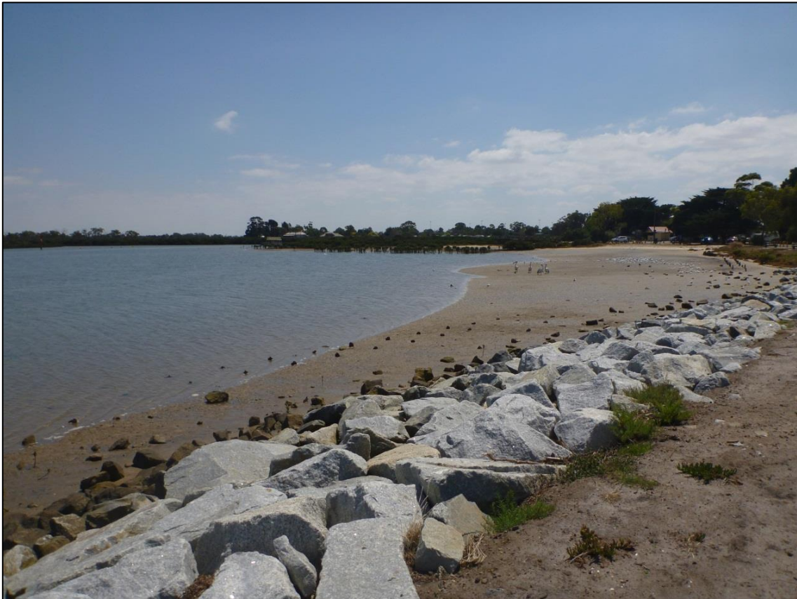
Figure 3-10 Rock Revetment Structure at Tooradin adjacent to Boat Ramp
