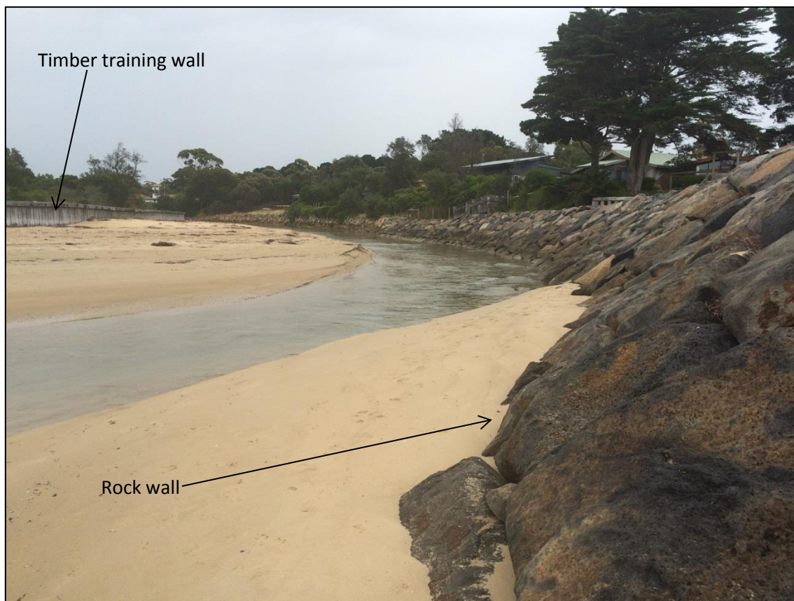
Figure 2-12 Merricks Creek Entrance Structures
