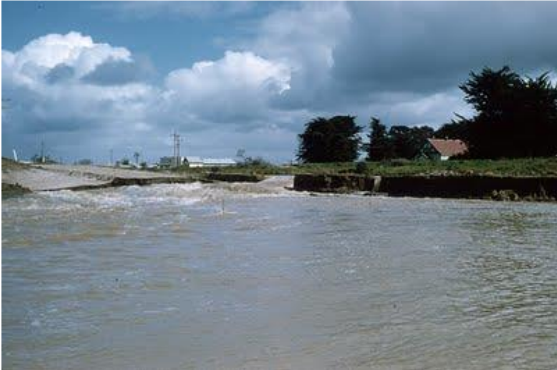
This photograph was taken by Jim Rouse, in October 1962, before the official opening of the Cora Lynn spillway. The building, with the brown coloured roof, is the Cora Lynn Hall. The other buildings you can see in the background are the same as the ones on the other Cora Lynn photograph at the
