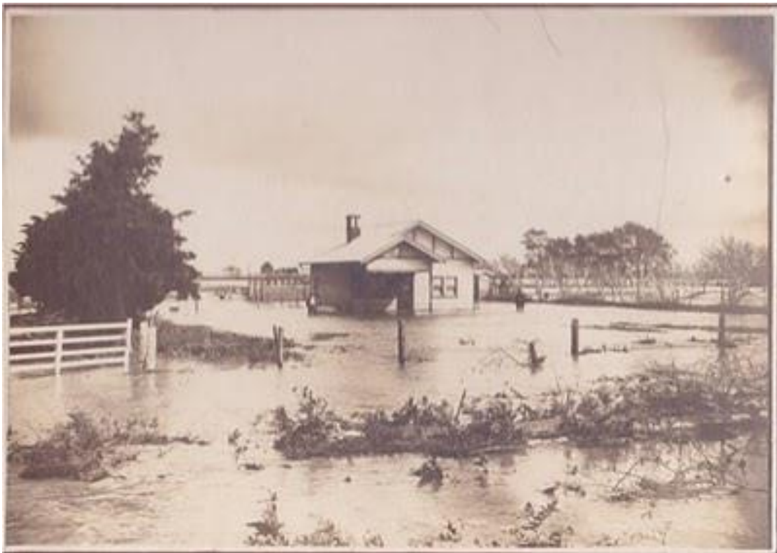
Corner of Main Drain Road and Dessent Road, under flood, in 1937
